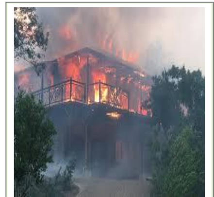
One of the properties damaged during the June 2017 Knysna and Plettenberg Bay fires, Western Cape fires.
